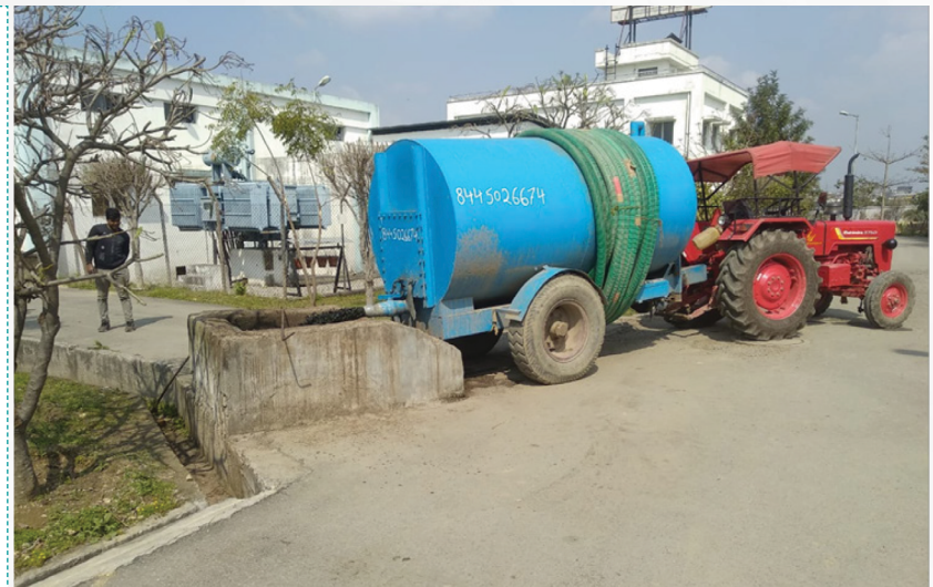
Current practice of direct discharge of FSS at inlet pumping station at Kargi Chowk STP
